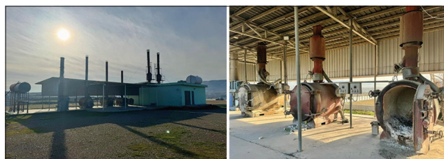
Fig. 8. Incinerators in the Tanjaro area.
