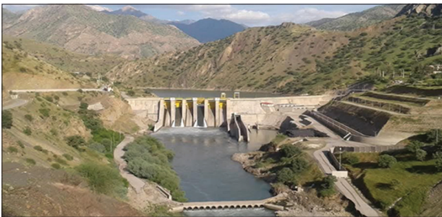
Fig. 7. Hirwa Dam looking upstream.
